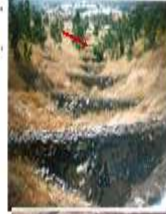
LOOSE BOULDER STRUCTURE
